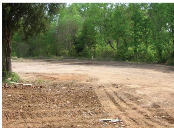
Arkwright Mill site after cleanup
